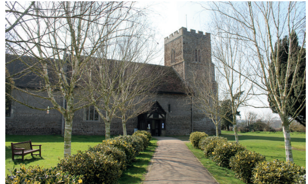
Figure 2 Photo of the Church of St Mary
